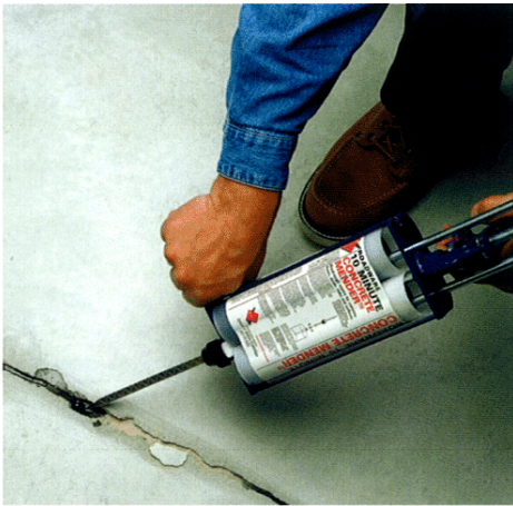
Roadware 10 Minute Concrete Mender™ is applied from self-mixing cartridges.
