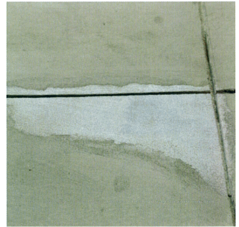
Repairs may be blended, polished, painted, or returned to traffic in just 10 minutes at 70° F!
